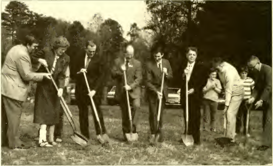
Participants in the Brandt Oaks groundbreaking on March 25, 1990 are (from l. to r.) Jim Clontz, Becky Newcomb, Jack Swanson, Ronny Reynolds of the Baptist State Convention's Church Extension Department, Dennis Blackmon of the Piedmont Baptist Association, Bob Clegg, Director of Church Building and Planting for the Baptist State Convention, Carl Myatt, and Fred Binder.
